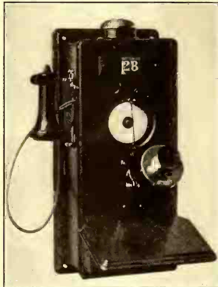
A Selective Calling Automatic Telephone for Farmers' Lines.
